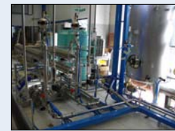
Section of nanofiltration and reverse osmosis
